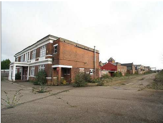
Facing South East
